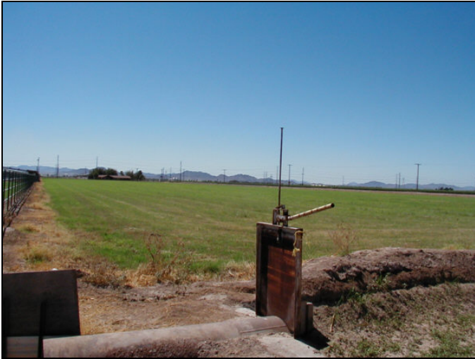
[4] NE Corner looking S
