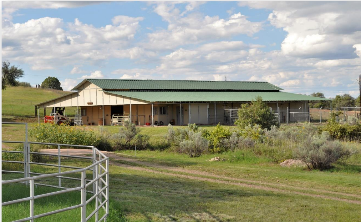
Custom Metal Barn with Turn-outs
