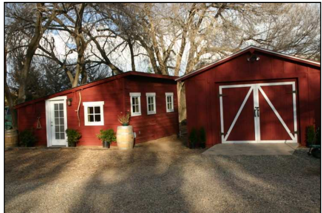
Winery Office & Cold Room
