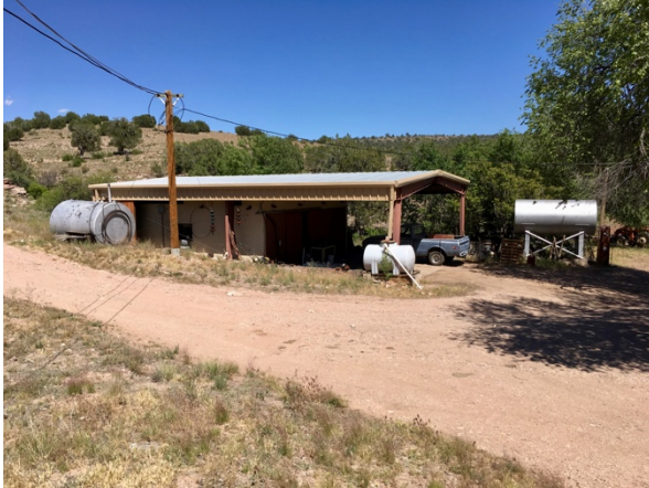
Shop and generator shed.
