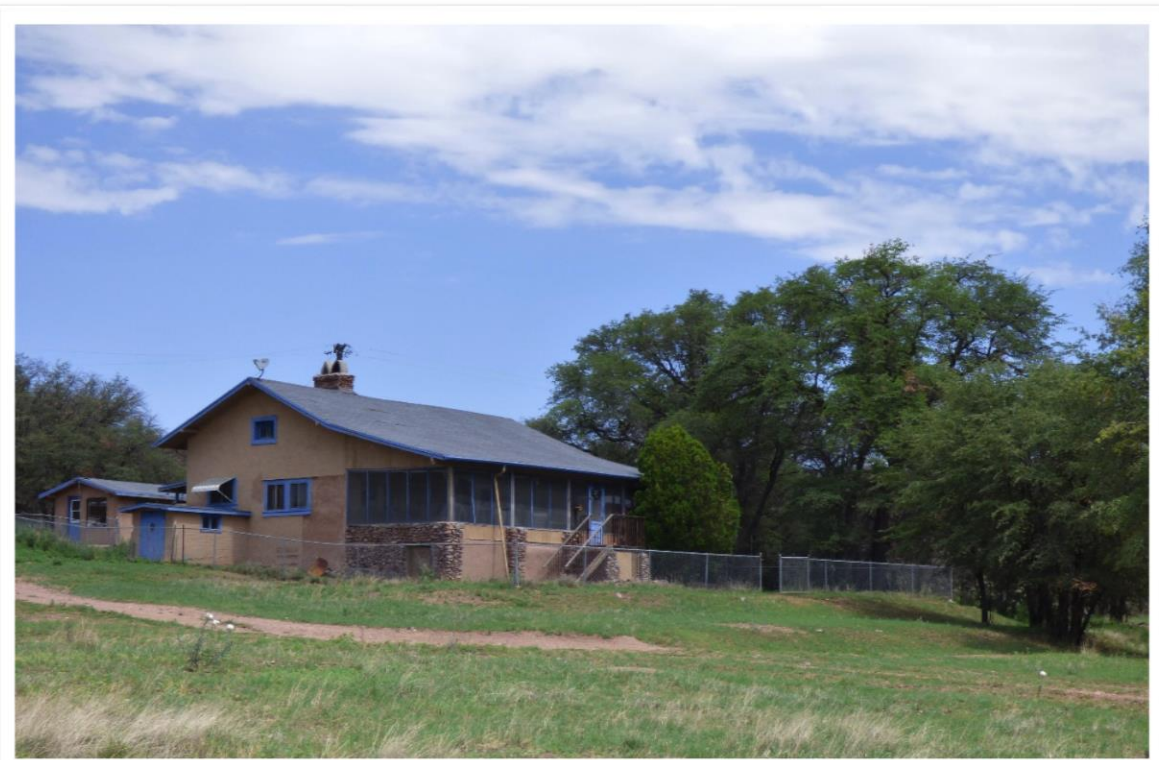
Historic Adobe Ranch House
